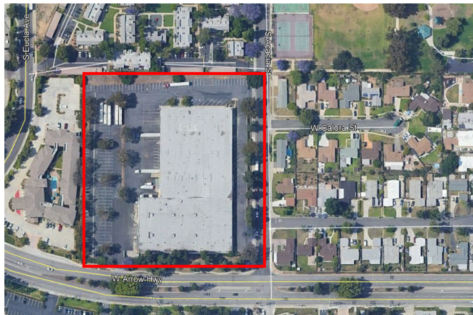
Figure A-8 Warehouse Site
